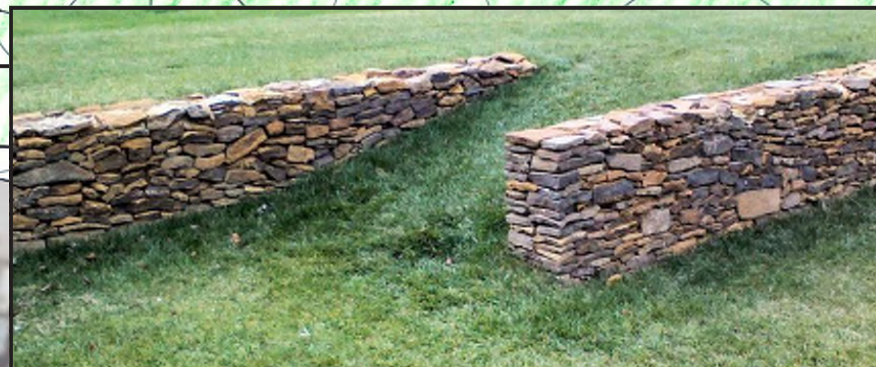
Stone Retaining Walls
